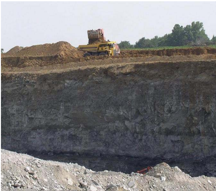
Surface soil is stripped off and stockpiled prior to coal mining.
